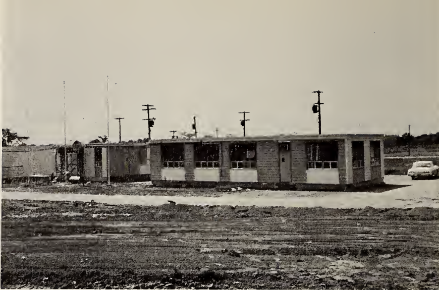
OLD CAMPUS SITE
